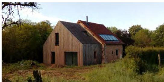
Guillet Ch. - Nodale V. architectes
